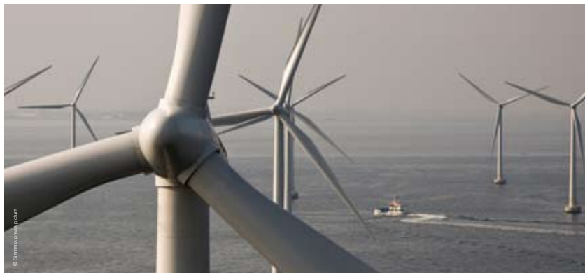
Offshore wind farm Lillgrund in the Øresund between Malmö and Copenhagen
