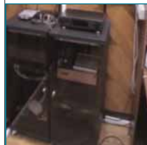
Rack Sala Senatului Senat Hall - Rack for equipments
